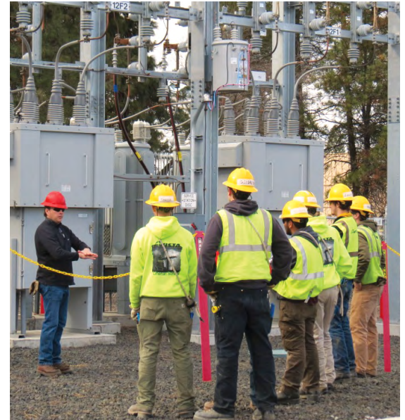
Avista Lead Line instructor Bill Magers gives a safety overview of working within an energized substation.
